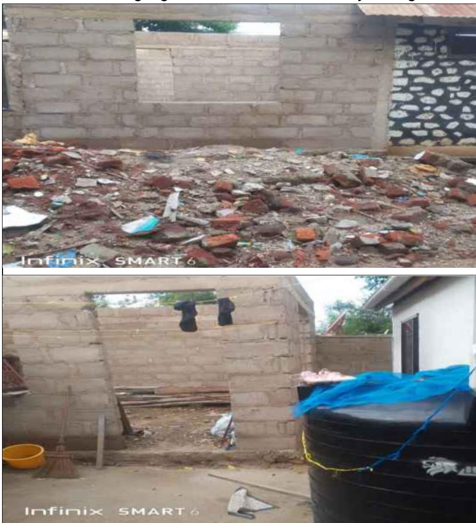
Photo 3.1: Ongoing Construction of Health Facility at Pangani
